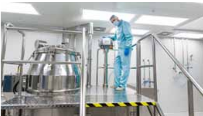
Plenum Access Lighting
